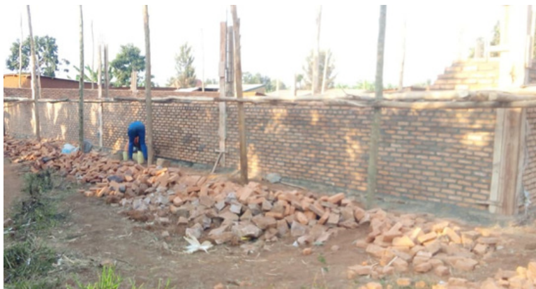
Construction of the COCURIKA Cooperative storehouse is progressing under the KIIWP II Matching Grant Scheme.
