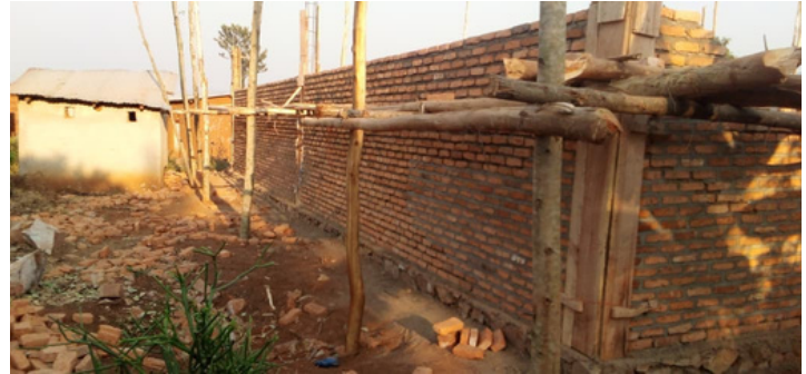
Steady progress in the construction of the COCURIKA Cooperative storehouse under KIIWP II.
